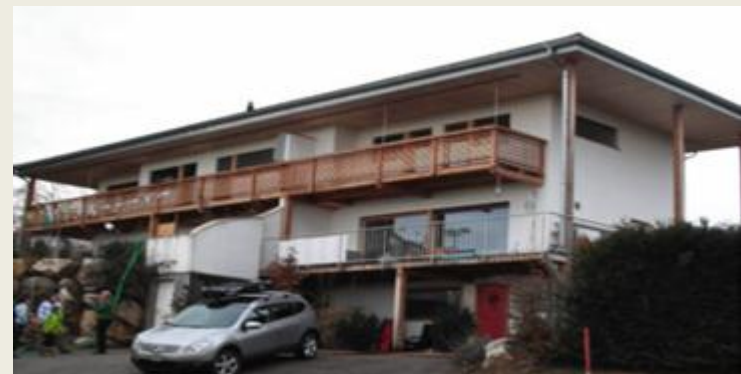
HEMP HOUSE Switzerland
